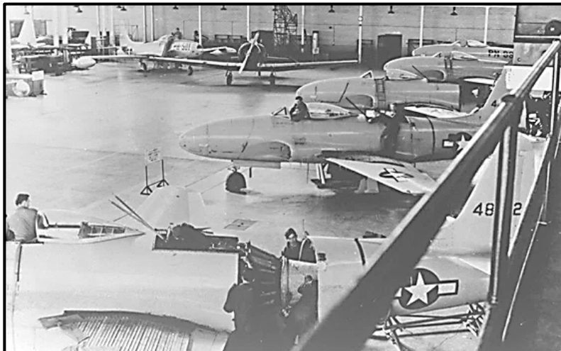
Airplane and engine mechanic jet propulsion generalized training began at Chanute. In this photo, students change an engine in an F-80-type plane.
