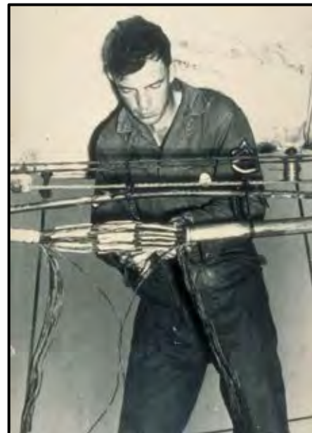
Scott Field – In the Cable Maintenance course, a student practices splicing techniques
